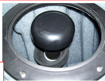
Float Shutoff Assembly
